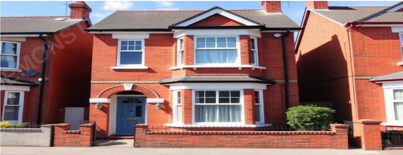
Front elevation photograph of the property
