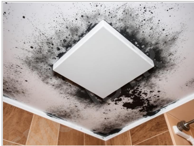
Photo 1 — First Floor Bathroom
